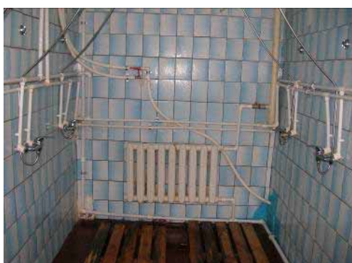
The repair works have been done with quality
