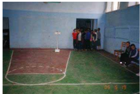
The sport hall before repair works
